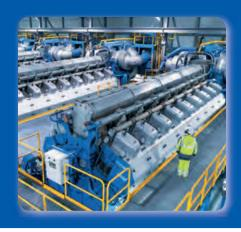
The Kiisa emergency reserve power plant in Estonia was commissioned by the national transmission system operator and operates only in case of a network failure or capacity shortfall. The plant reaches 100% load in less than 10 minutes, can operate with different fuels and down to a bonechilling -80°C, securing the national electricity supply.
